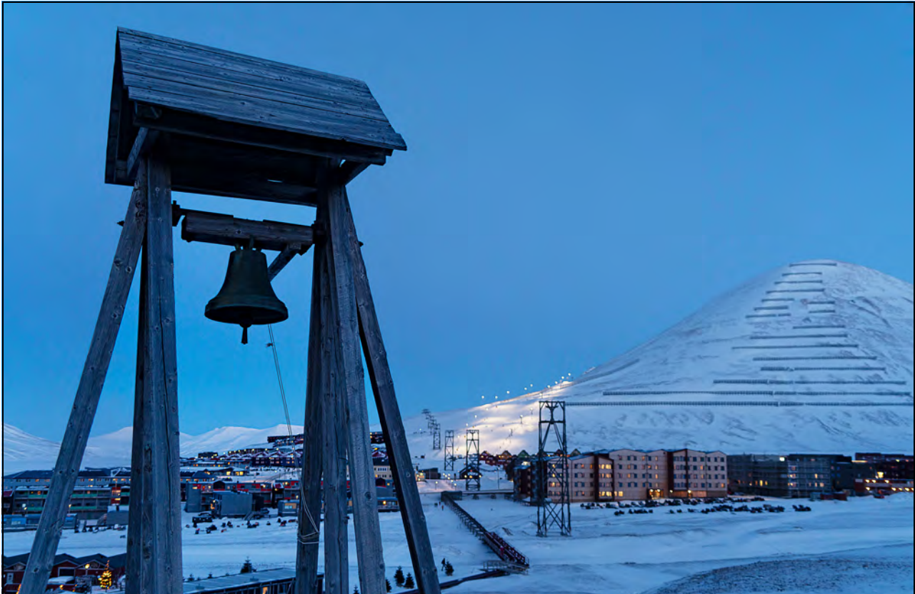
Figure 4.1 View from Skjæringa towards the town centre with avalanche barriers and slalom slope in the background.
