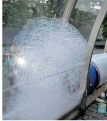
2. Insulation with soap bubbles.
